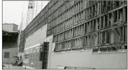
After the 1975 season, the original tin facing of the Green Monster was stripped off.
